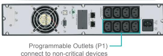
Programmable Outlets (P1) connect to non-critical devices
